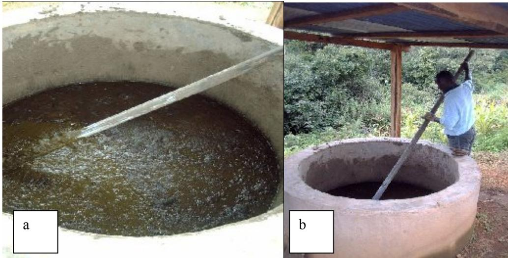
Figure 10(a&b). Biogas mixing tank with fresh cow dung
