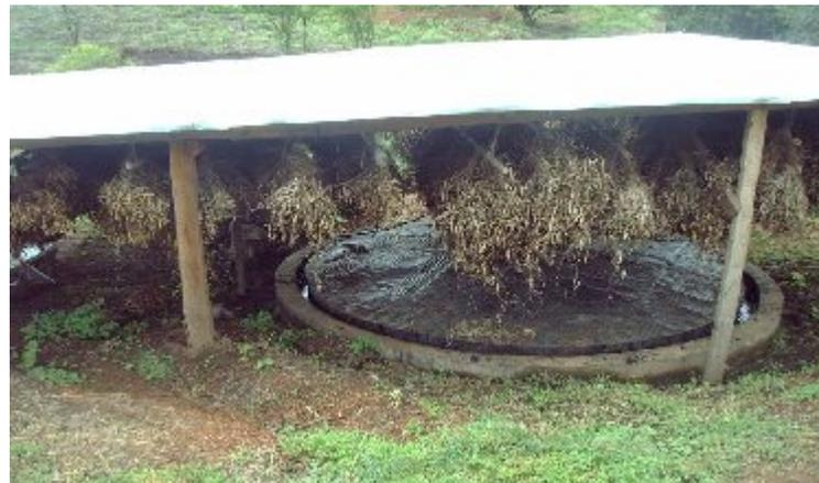
Figure 11. Inverted drum on digester with no biogas
