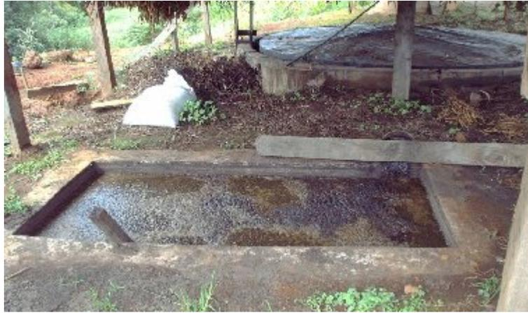
Figure 13. Biogas by-product (slurry) tank
