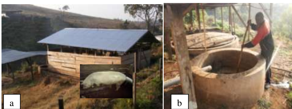
Fig.8. Obtaining pig dung for biogas production.a: BIOFARM piggery attached to the biogas system; b: biogas plant mixing tank.
