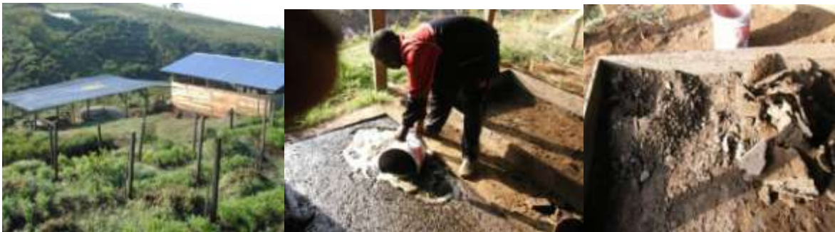
First picture present biogas system linked to piggery, second biogas slurry being removed from its chamber and third dried biogas slurry
